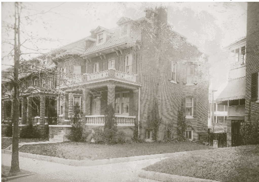
Rowhouses at 3664-3674 Park Place and at 608 Rock Creek Church Road, ca. 1920.
